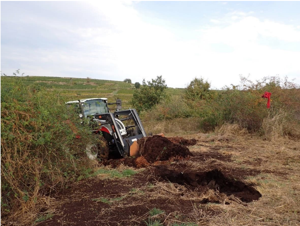
Entfernung der illegalen Treberdeponie 14.10.2023 (B. Thurner)
